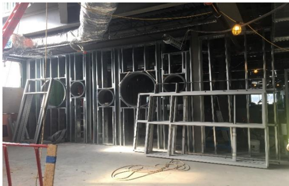
Interior steel stud framing in the 2 nd /3 rd grade wing is now finished, and the hollow metal borrowed lights have now been framed; we will be hanging dens board in this area in the coming weeks.
