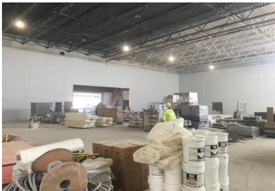
Inside the gym, the painters are busy coating the precast walls and joists with primer, and then they will paint the final color!
