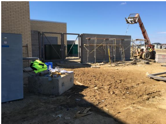
The masons are laying block for the garbage enclosure that is behind the kitchen. Once that is complete, all of the block for the school will be installed!
