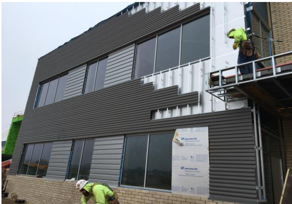
The metal panels are being put up very quickly. As seen in this photo, they are attached to the building via a rail system that was installed earlier.
