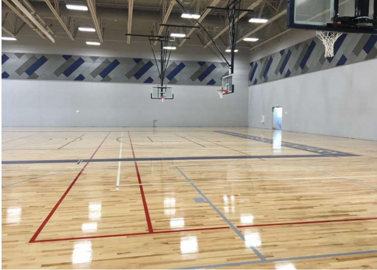
The gym floor is painted and polished! It will be ready for use by the end of next week after it dries.
